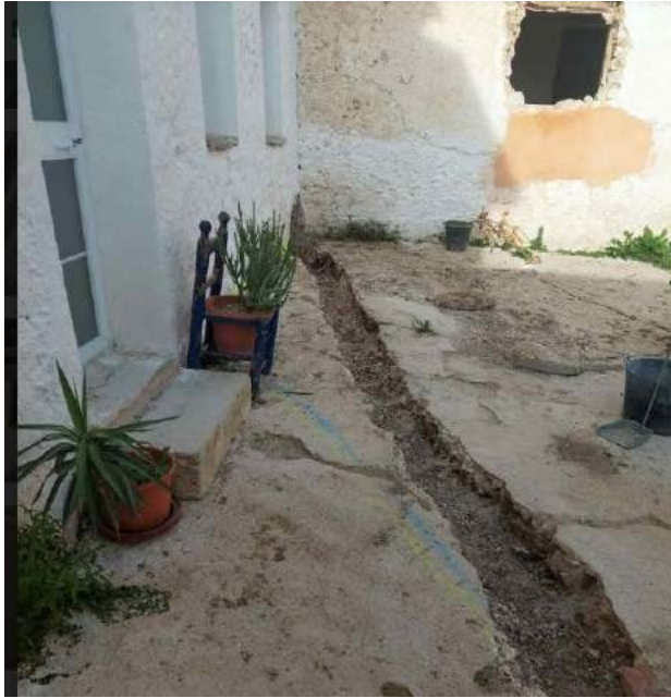
On the left channels already made in the courtyard going to the new kitchen and on the right channels and progress in the dining room.
